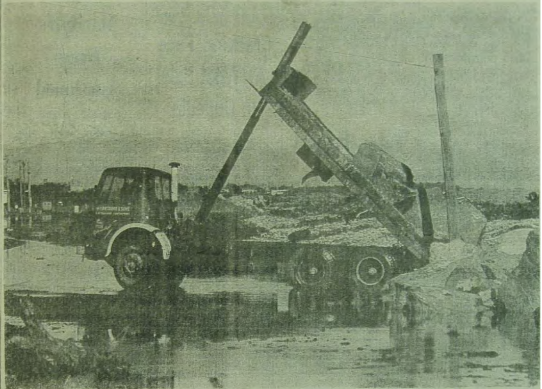
Rock was rushed to the scene of a breach in the sea wall at Dommert
