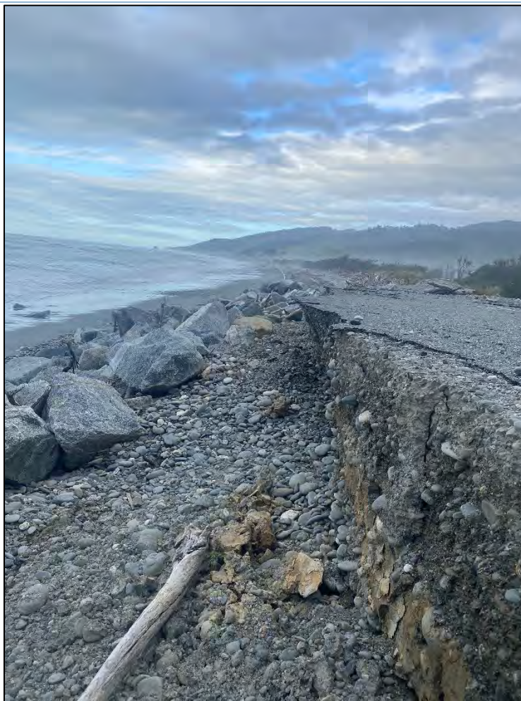
Figure 2-4 – Severe erosion of wall, with rock protection falling away from the wall completely
